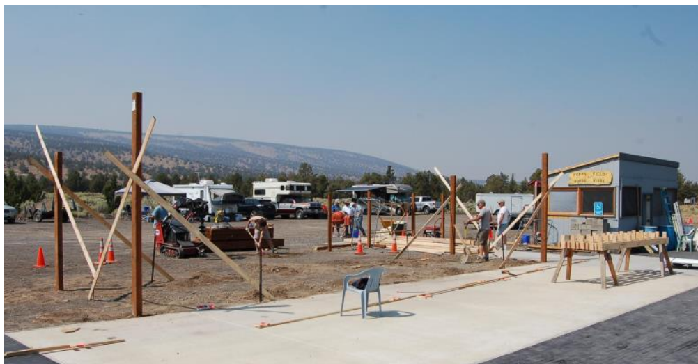
Construction work begins on the eastside shade structure.
