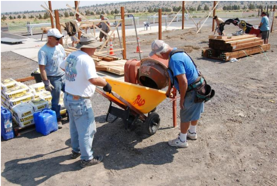
Joe Newman, Chris Shaker and the Dave Reiss (aka The Boss) mix concrete for all of the shade structure post holes.
