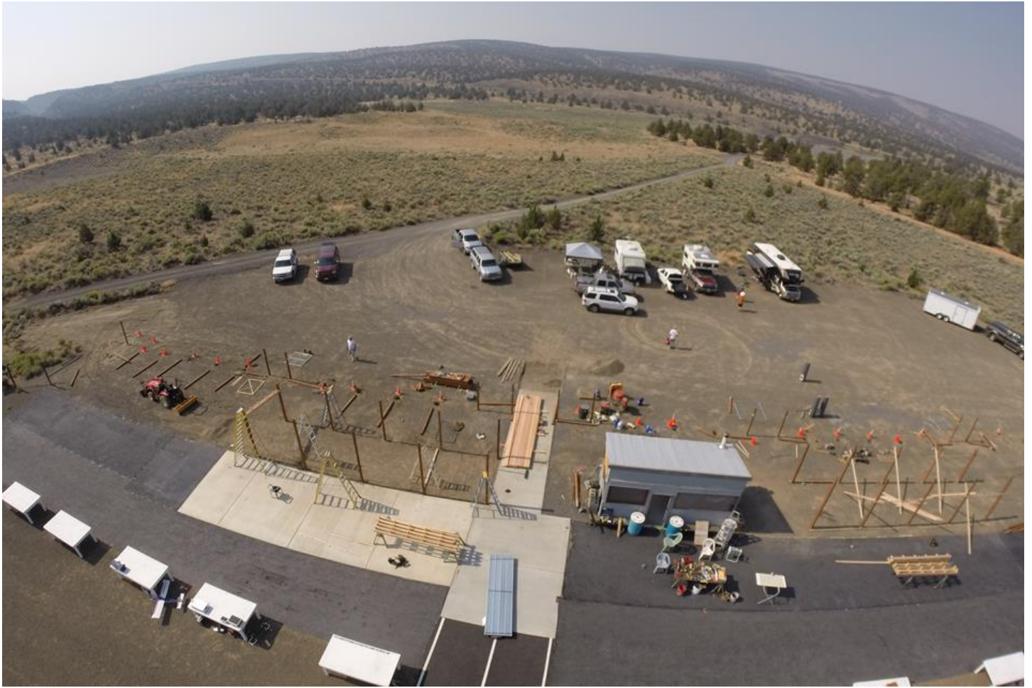
An aerial view Popp's Field during the construction phase of our project.
