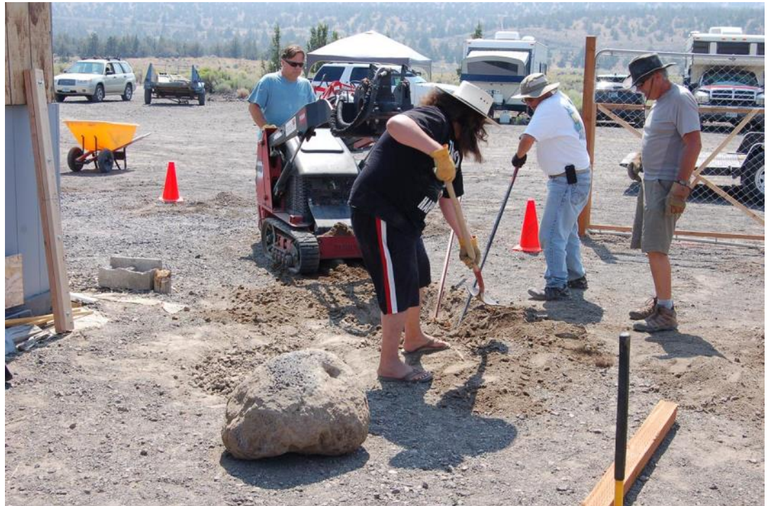
Galen Ruud, Kurt McNutt, Chris Shaker and Mike Dressler fill in the hole that this 300lb rock occupied for centuries. This rock was responsible for tripping many of our pilots and guests over the years. Fair well you old rock!
