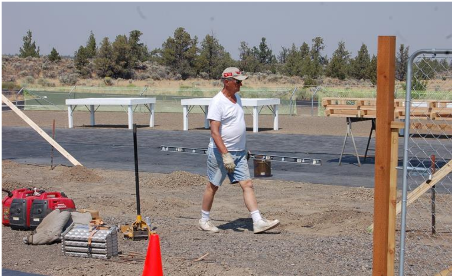
Inspector Schramm carries his level for a surprise inspection on the east shade structure. Tom kept us on our toes all week with surprise inspections. We did well because no citations were issued during the week.
