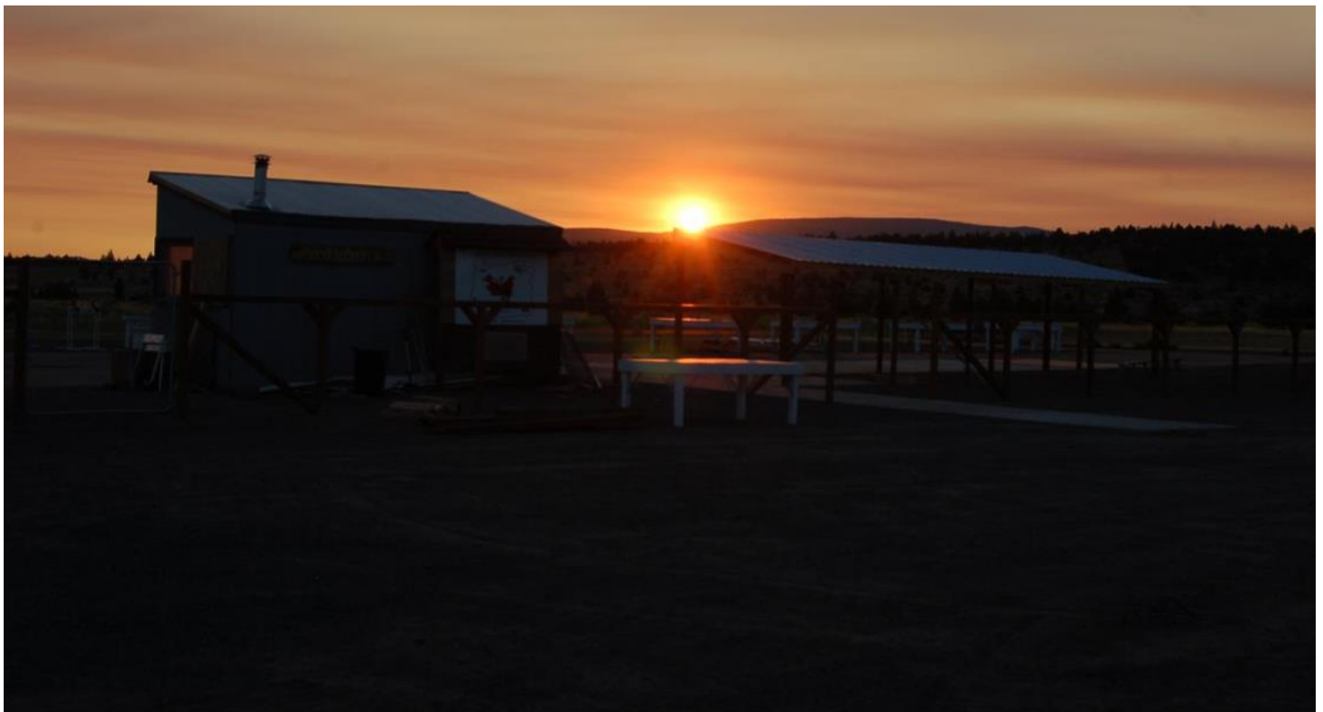
The dawn of the first day following the completion of the BAM Shade and Fence Project.
