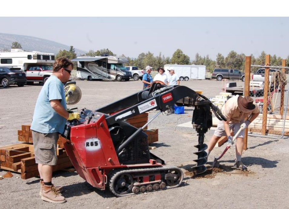
Galen Ruud and Mathew Phillips drilling post holes for our new fence.
