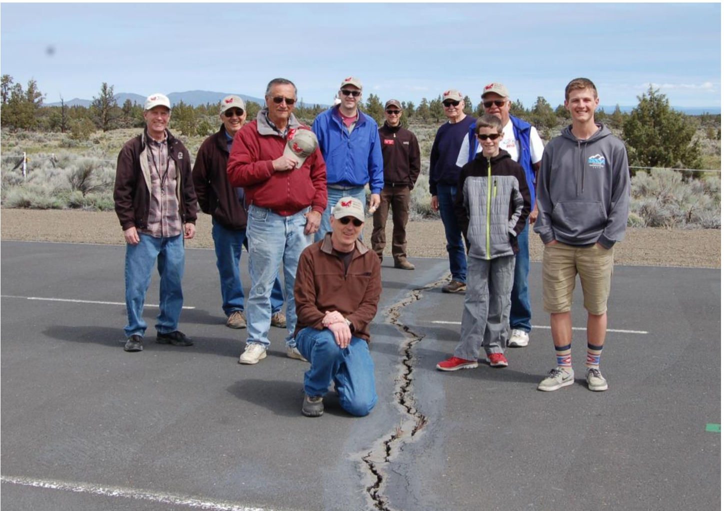
Saying “goodbye” to those nasty runway cracks are: (from left to right) are Richard Carlson, Jon Putnam, Tom Schramm, Waldemar Frank, Larry Vose, Tom Rose, RJ Gorman, Dave Reiss, Brian Downer and Chris McDougal (kneeling).
