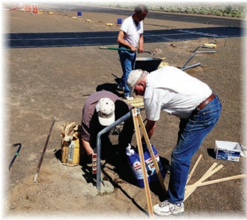
The actual mixing of the concrete was done in the holes.
