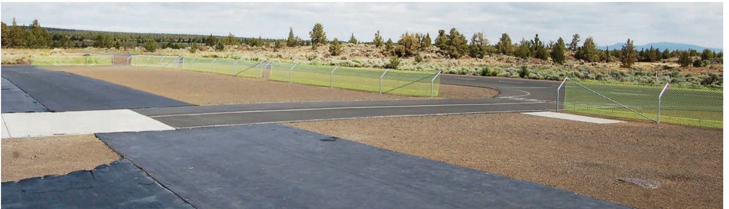
Braces were installed and the top cable was then stretched through the drilled holes and the fabric was hung. On the bottom of the fabric, re-bar was installed to weight the fabric. The finishing touch came in the form of caps for each post.
