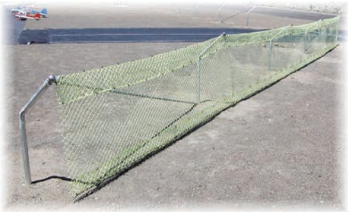
Braces were installed and the top cable was then stretched through the drilled holes and the fabric was hung. On the bottom of the fabric, re-bar was installed to weight the fabric. The finishing touch came in the form of caps for each post.
