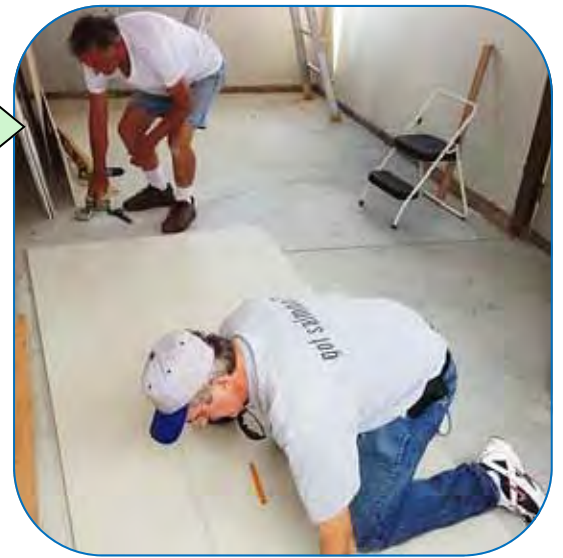
Greg McNutt measuring and cutting a whole lot of insulation. He installed most of it himself .
