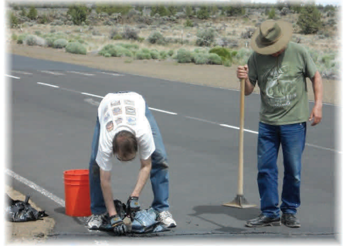
Two Members repairing one of the cracks in the runway.
